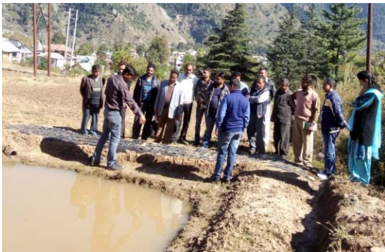
Showing newly constructed IFFU to field functionaries
